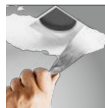
skimmed into plasterboard ceiling (trimless)
