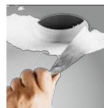
skimmed into plasterboard ceiling (trimless)
