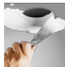
skimmed into plasterboard ceiling (trimless)
